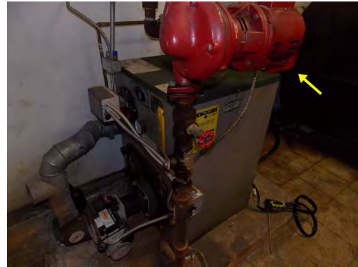
This oil-fired hydronic boiler serves the entire development. Also shown is the circulating pump.
