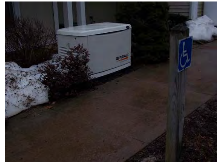
This propane-powered generator provides 17 kW of emergency power.
