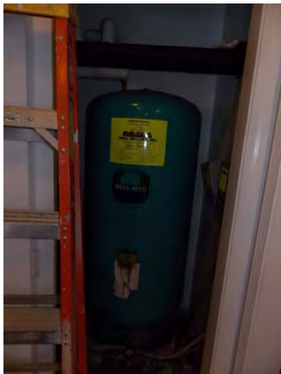
This is the well water pressure tank.
